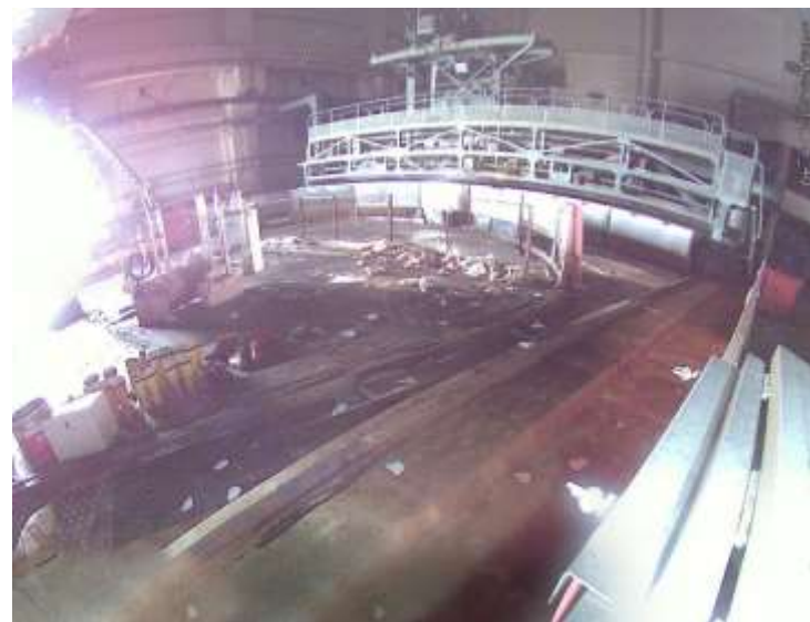
Unit 2 Operation floor
